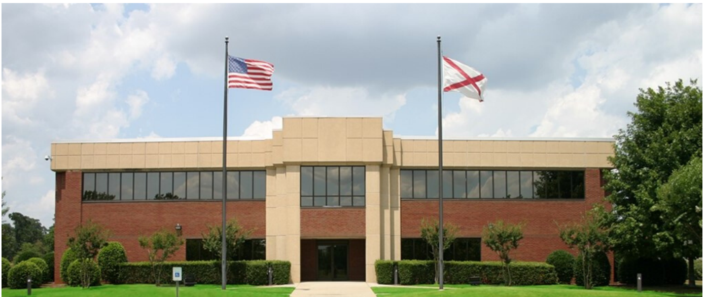
Alabama Supercomputer Authority Data Center, Huntsville, Alabama
